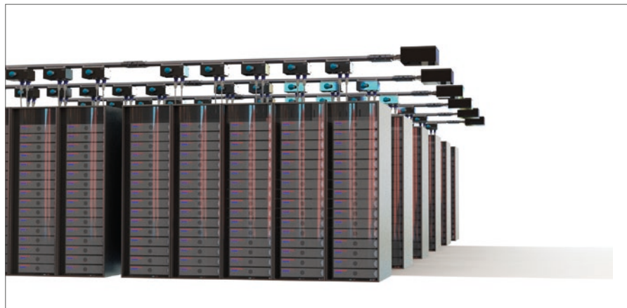
'Hot Aisle Cold Aisle' Arrangement
