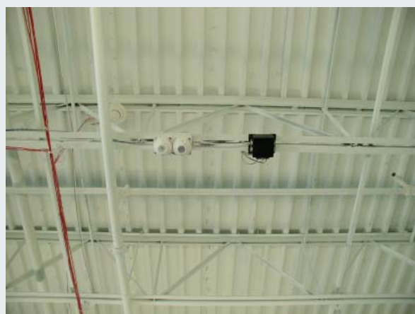
Figure 16. SensorSwitch daylight, occupancy sensors
