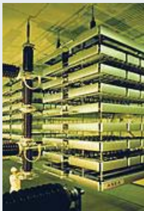
Figure 2. HVDC thyristor valves
