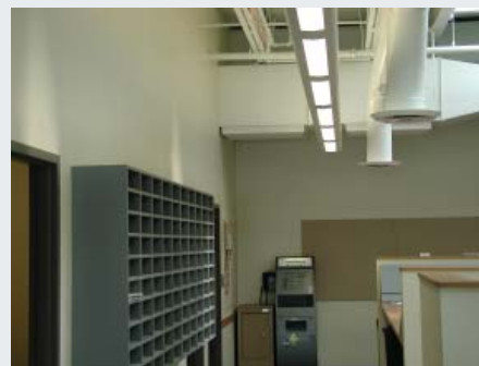
Figure 15. Office and warehouse lighting systems use DC power
