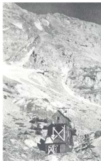
Figure 24. The first AC generation plant, Ames, Colorado
